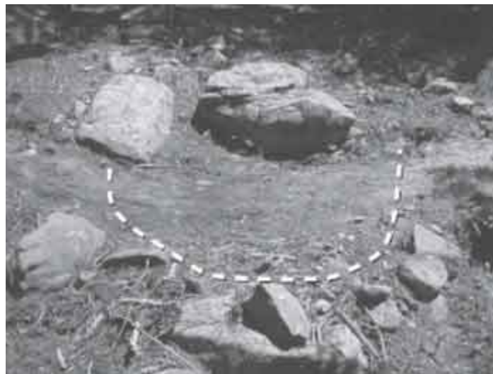
Figure 13 – Knicks constructed into existing trails will drain puddles from flat areas.
