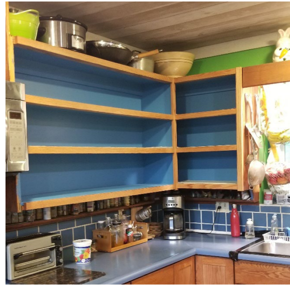
Shelves braced with 1x2 oak in three directions
