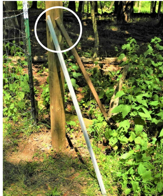
Placing the First Post. Braced to vertical.
